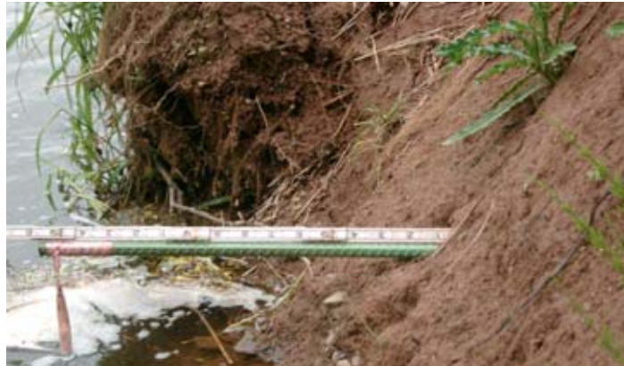
Figure 6.2 Measuring erosion loss using the bank-pin method at cross-section 53 just upstream of Delhi.
