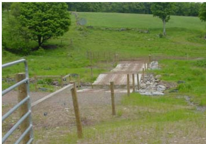
Figure 6.10 Fenced livestock crossing with animal walkway.
