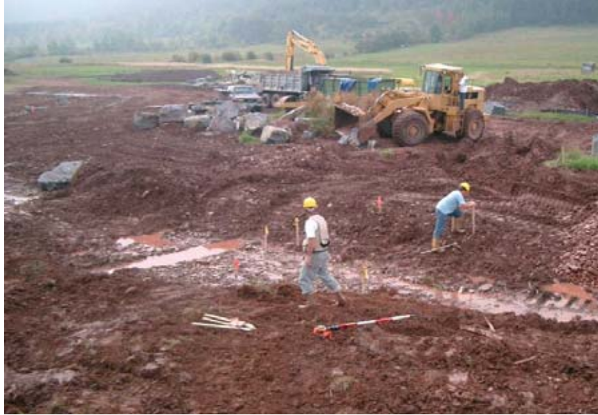
Figure 6.16 Photo taken during construction showing newly excavated channel and layout for a vane structure.
