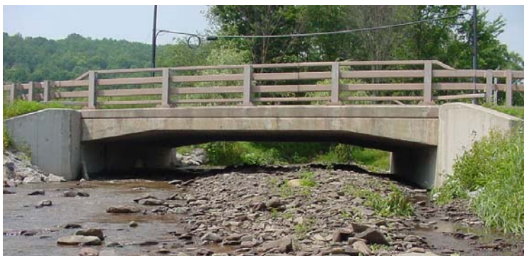
Figure 2.5 Gravel deposit under McMurdy Brook bridge on NYS Route 10 near Hobart. Note restriction of the waterway.
