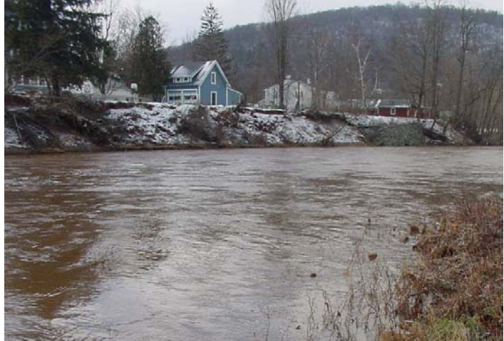
Figure 2.8 South Street location showing condition of embankment (December, 2000).
