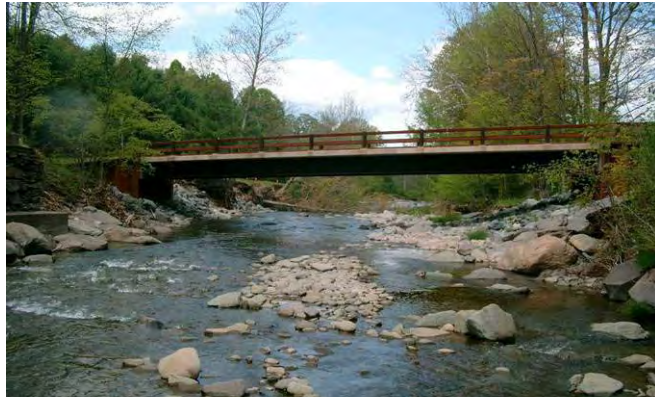
Figure 3.14 Bridge at Erpf Road
