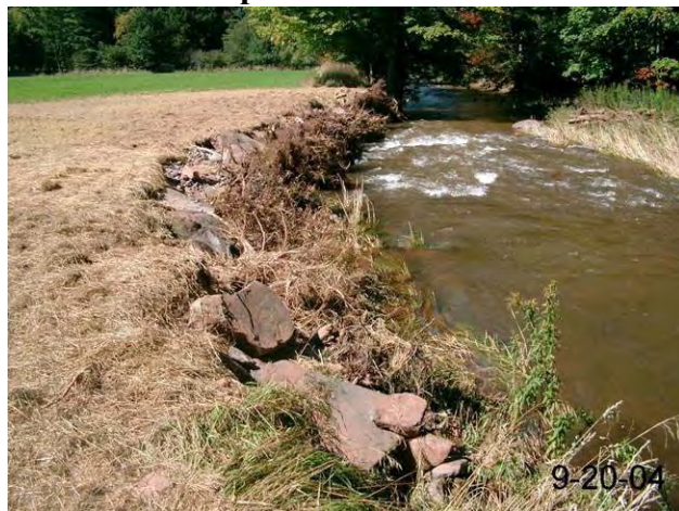
Figure 3.18 Root wad Installation Taken After the September 18, 2004 Storm
