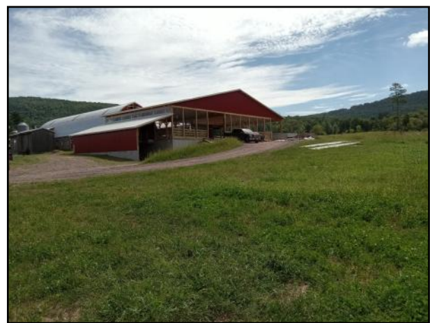
Byebrook before retractable curtain installed.
